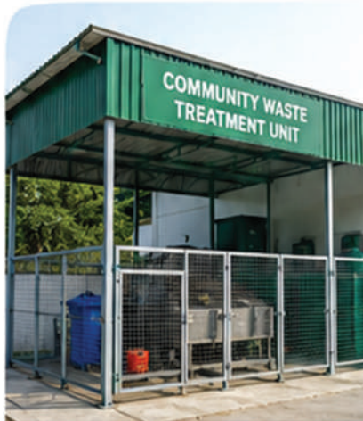
Community Waste Treatment Units
